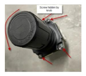
2. Remove adjustment knob and spring to expose the diaphragm seal
